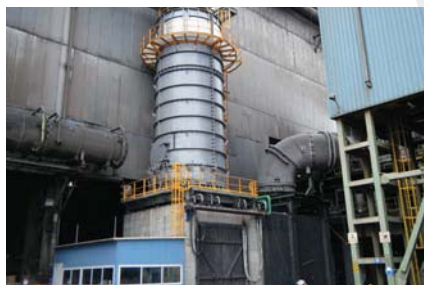
Compact arrangement of HTQ components: inlet duct (right), cooling tower and valve rack (behind blue housing)
