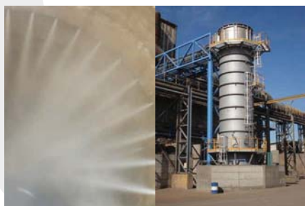
Compact arrangement of HTQ components: inlet duct (right), cooling tower and valve rack (behind blue housing)
