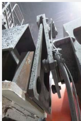
Simple mechanical solution with special plates mounted on the tool to be used (left side) and robot arm (right side)
