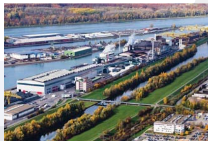
BSW mini-mill in Kehl / Germany – an example for operational and cost efficiency
