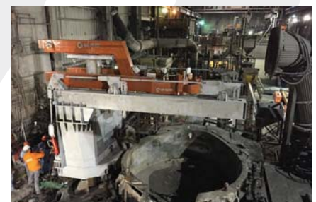
Installation of components at ASA site
